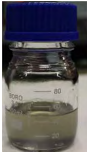
Figure 47: Oil drained from refrigerant circuit after 30 min of operation of compressor no. 2
